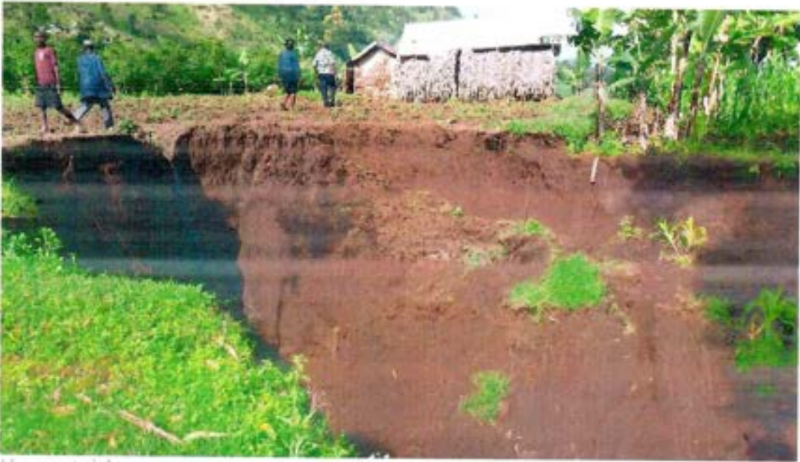
House at risk
