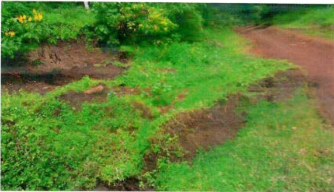
Figure 1: Soil block that is creeping (slow movement that results into a landslide) in Bulambuli District
