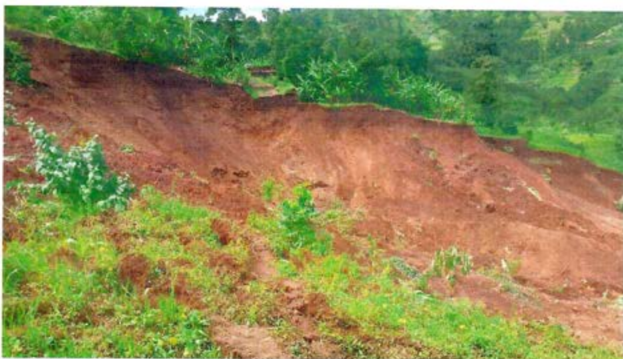
Buwangani to Shikunga road was cut off
