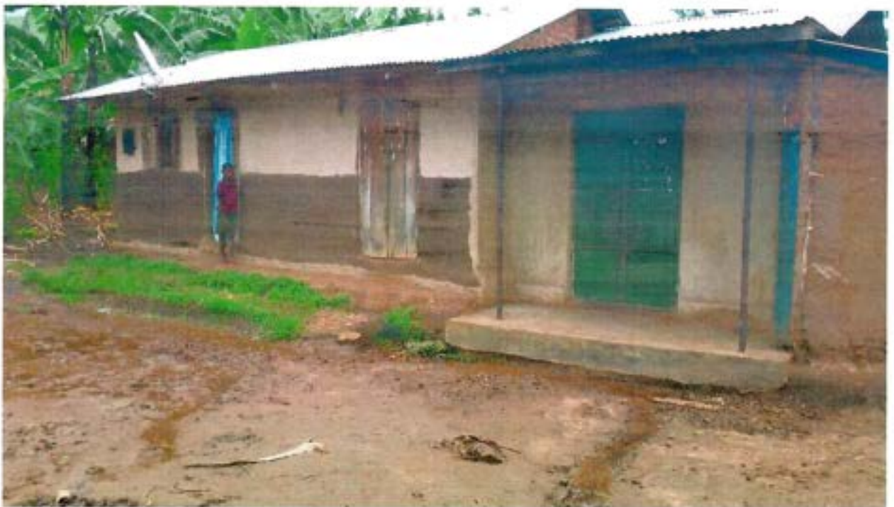
Water emerges from people's houses after landslide occurrence
