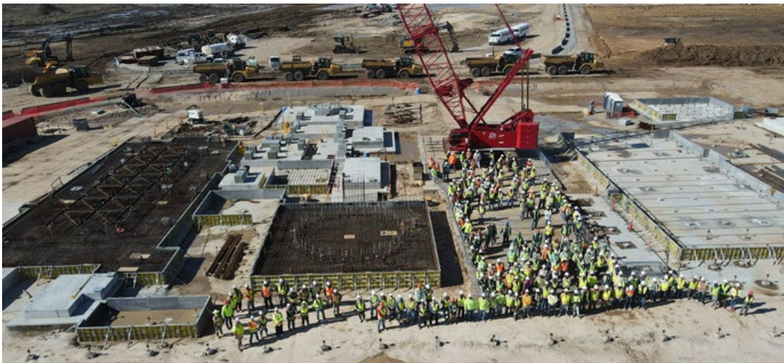
Figure 1. January 2023 photo of construction progress at Driftwood Terminal Site 1
