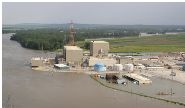
Figure 22.5: Floodwaters from the Missouri River surround the Omaha Public Power District’s Fort Calhoun Station, a nuclear power plant just north of Omaha, Nebraska, on June 20, 2011. The flooding was the result of runoff from near-record snowfall totals and record-setting rains in late May and early June (NWS 2012). 115 A protective berm holding back the floodwaters from the plant failed, which prompted plant operators to transfer offsite power to onsite emergency diesel generators. Cooling for the reactor temporarily shut down, but spent fuel pools were unaffected. 116 Photo credit: Harry Weddington, U.S. Army Corps of Engineers.
