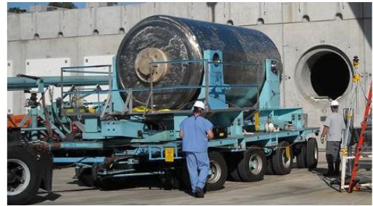
Workers prepare to load an AREVA-TN NUHOMS canister into a concrete storage module at the Calvert Cliffs Nuclear Power Plant in Lusby, MD. (Courtesy: Exelon)
