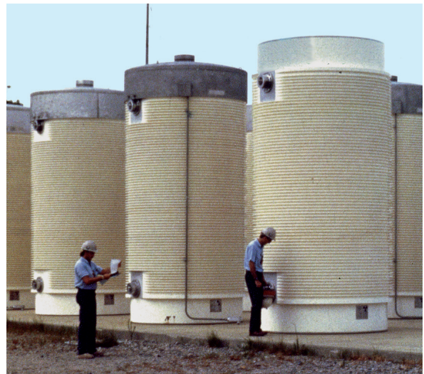
Inspectors examine dry storage casks containing spent nuclear fuel.
